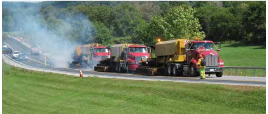
WAITSFIELD / MORETOWN. Paving project.
